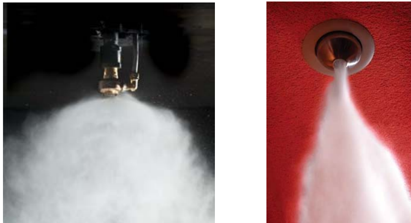
Figure 1: Two examples of hybrid water mist systems currently on the market. (left) Victaulic Vortex system discharging. (right) ANSUL Aquasonic system discharging.
